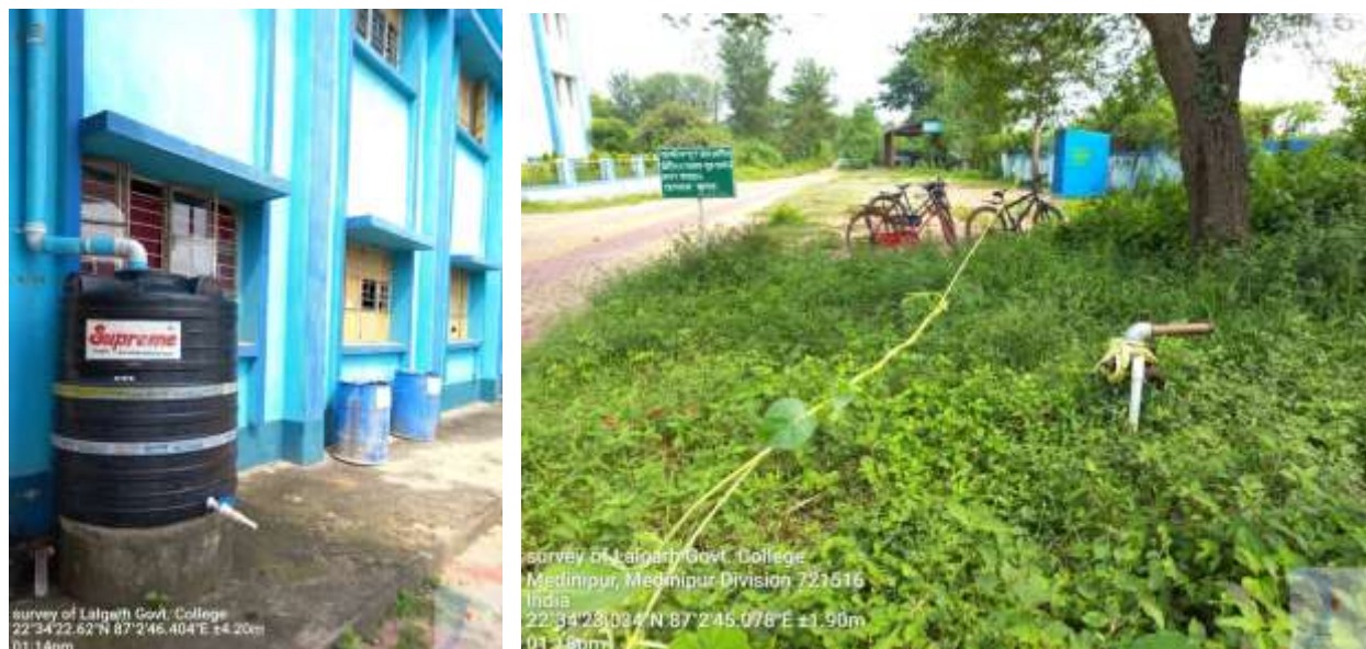
Rainwater harvesting site in the college premises
